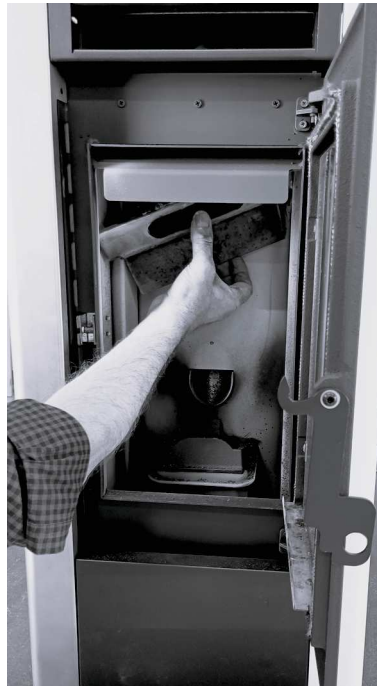
Fig. 23 - Remove the head of the firebox 2
